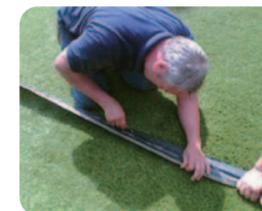
step2: Cutting the grass edges to fit the field size before you glue the seams.
