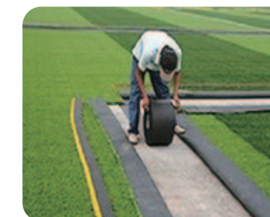
step3. Joining the tape in place.
