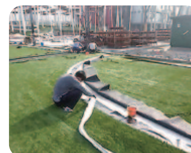
step7: Putting the white grass in the right place.
