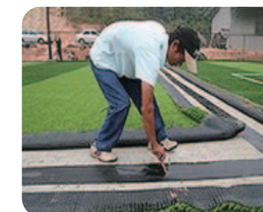
step6: Brushing glue on the tape and the edges of two grass carpet.
