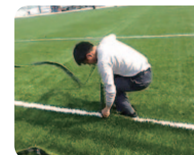
step8: Cutting the green grass which overlap on the white grass.
